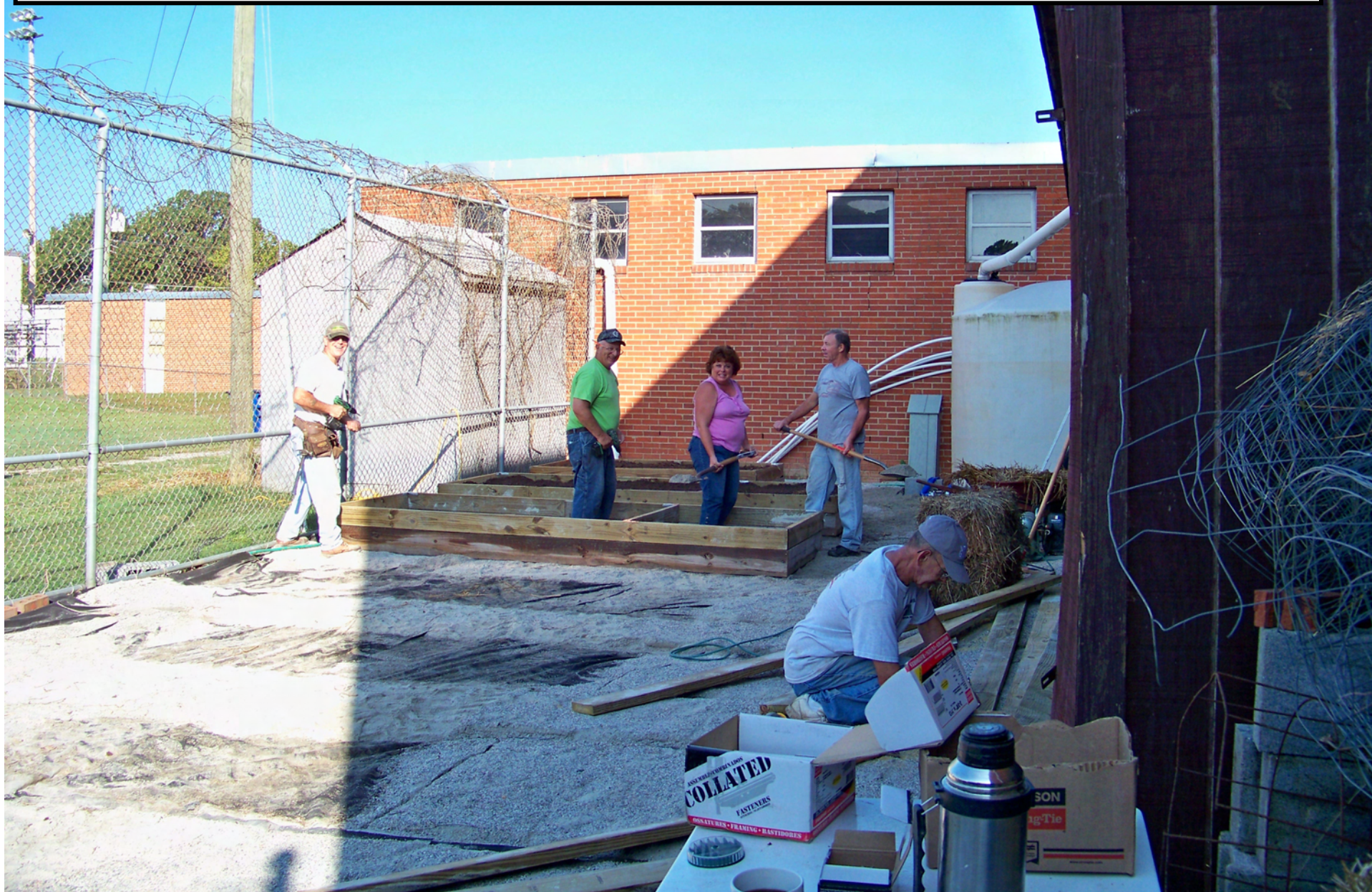
Construction of demonstration garden with help of Extension volunteers.
