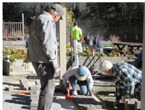
Pavers installing the patio
