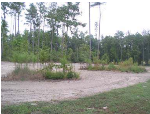
Area being cleared in Freedom Park.
