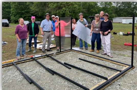
Greenhouse Construction Crew (Photo Courtesy of Bill Dichtel)
